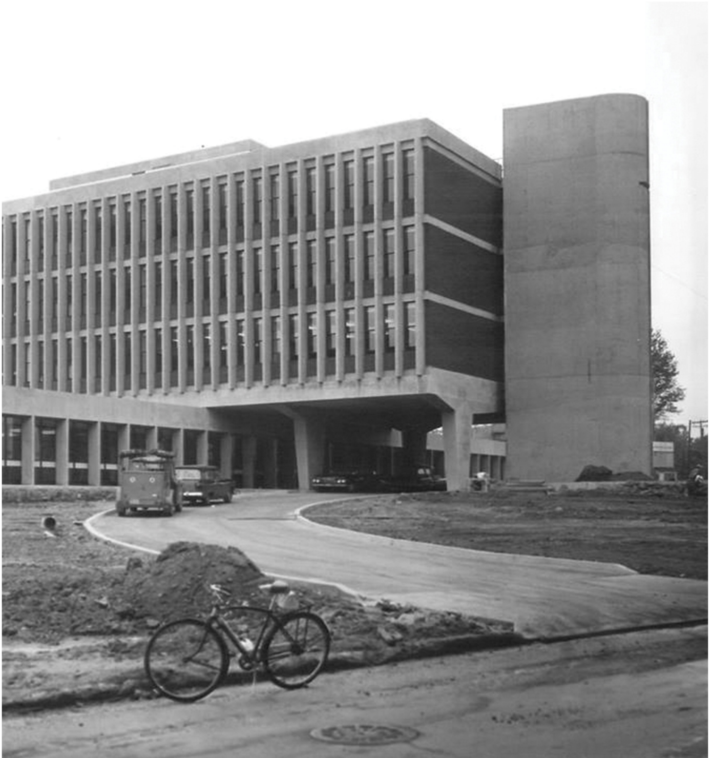
The construction of Monsignor Farrell High School
